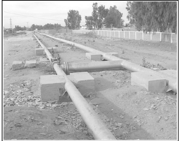
Open pipelines at Sui.
