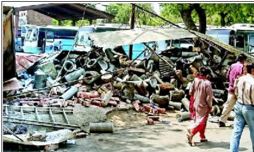
The aftermath of an encroachment demolition drive.
