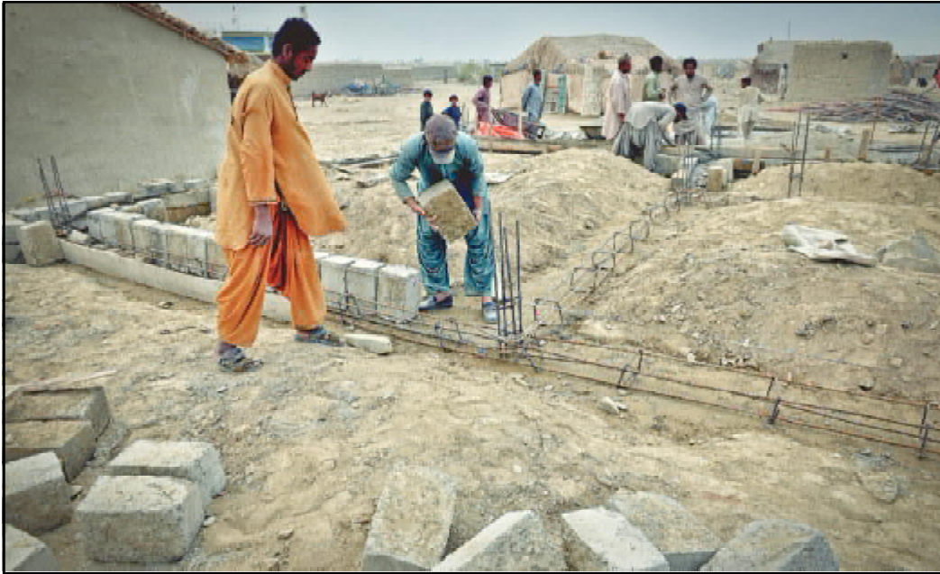
A labourer places a cement brick alongside an iron framework of a house that is being constructed in Malaar, Awaran. More than one year after the earthquake, reconstruction is still under way in the town.
