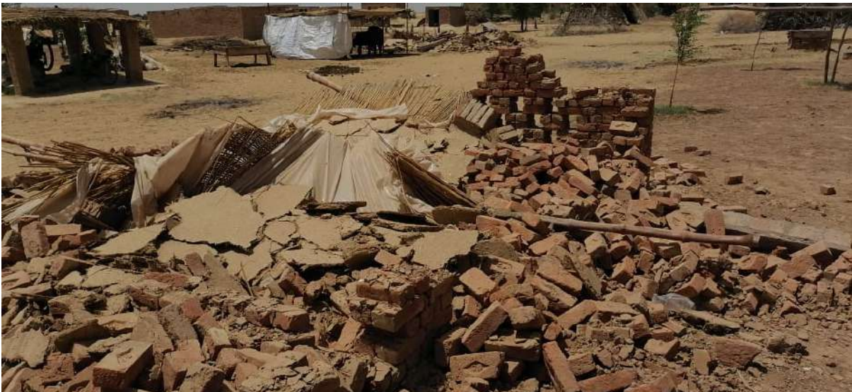
One of the houses in Chak 52/DB demolished by the local administration
