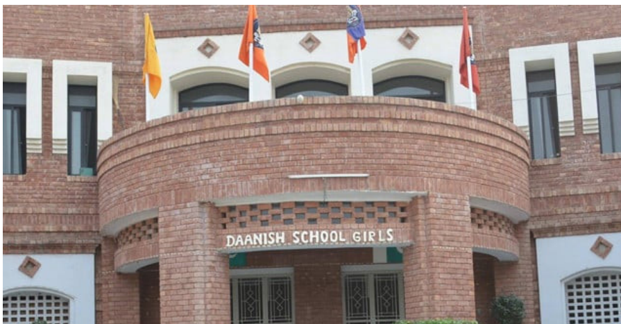
The construction on AJK's first Daanish School in Bhimber began in January.
