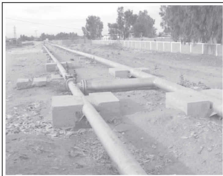
Open pipelines at Sui.
