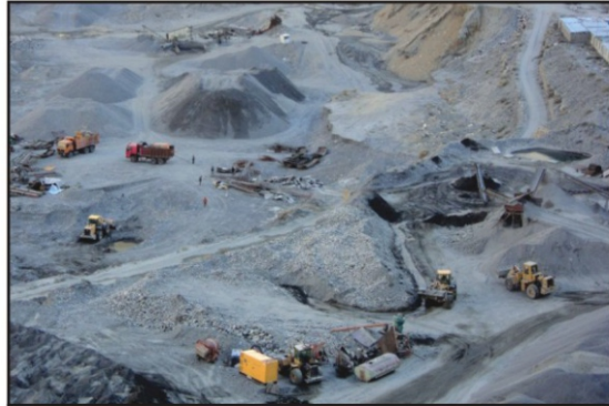
Efforts underway to restore the KKH link.
