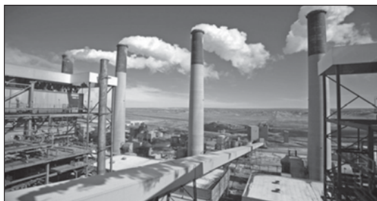
Coal-fired power plants are crucial to the CPEC project
