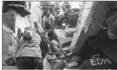
A three-storey dilapidated building in Karachi collapses and claims six lives
