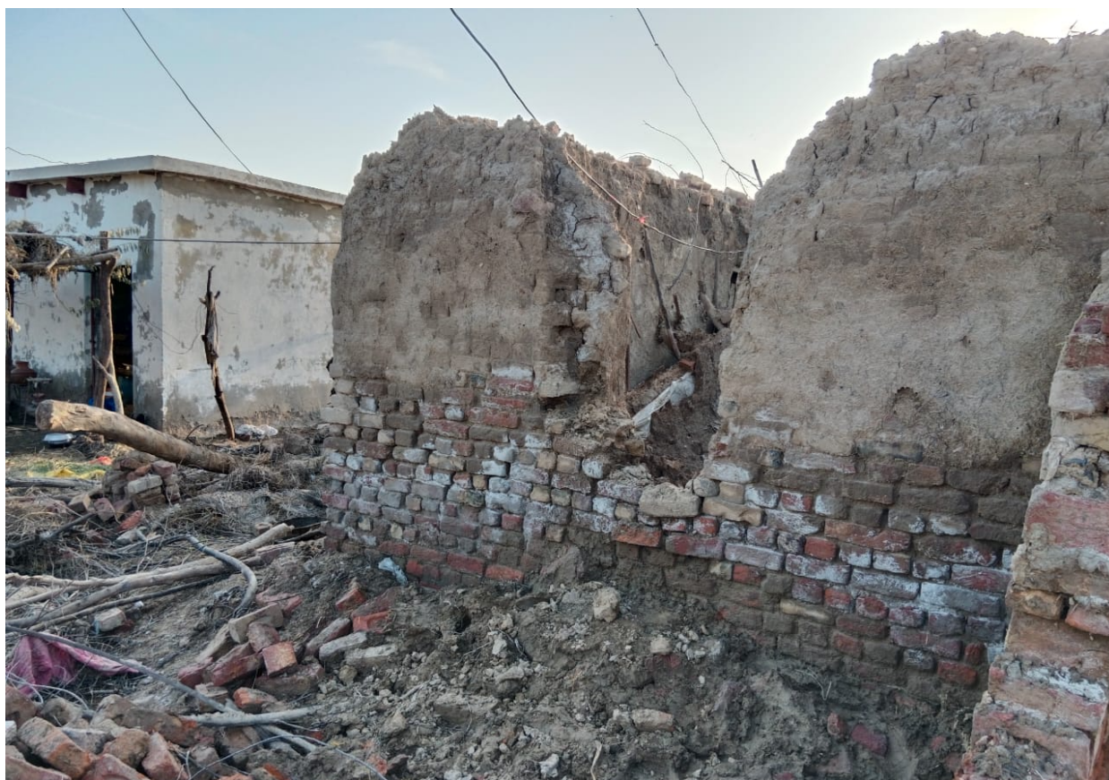
The scale of destruction to buildings meant that many survivors were forced to sit out in the open
