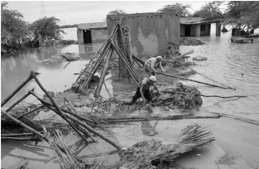
A large number of public and private properties and infrastructure were damaged during the mid-year flash floods.
